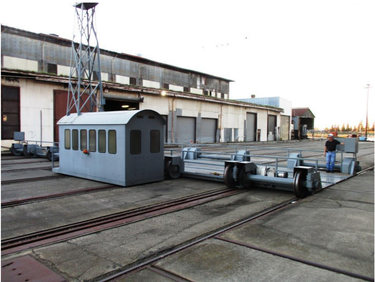
Mike H. tests the transfer table "bridge" after inspecting its structural integrity
