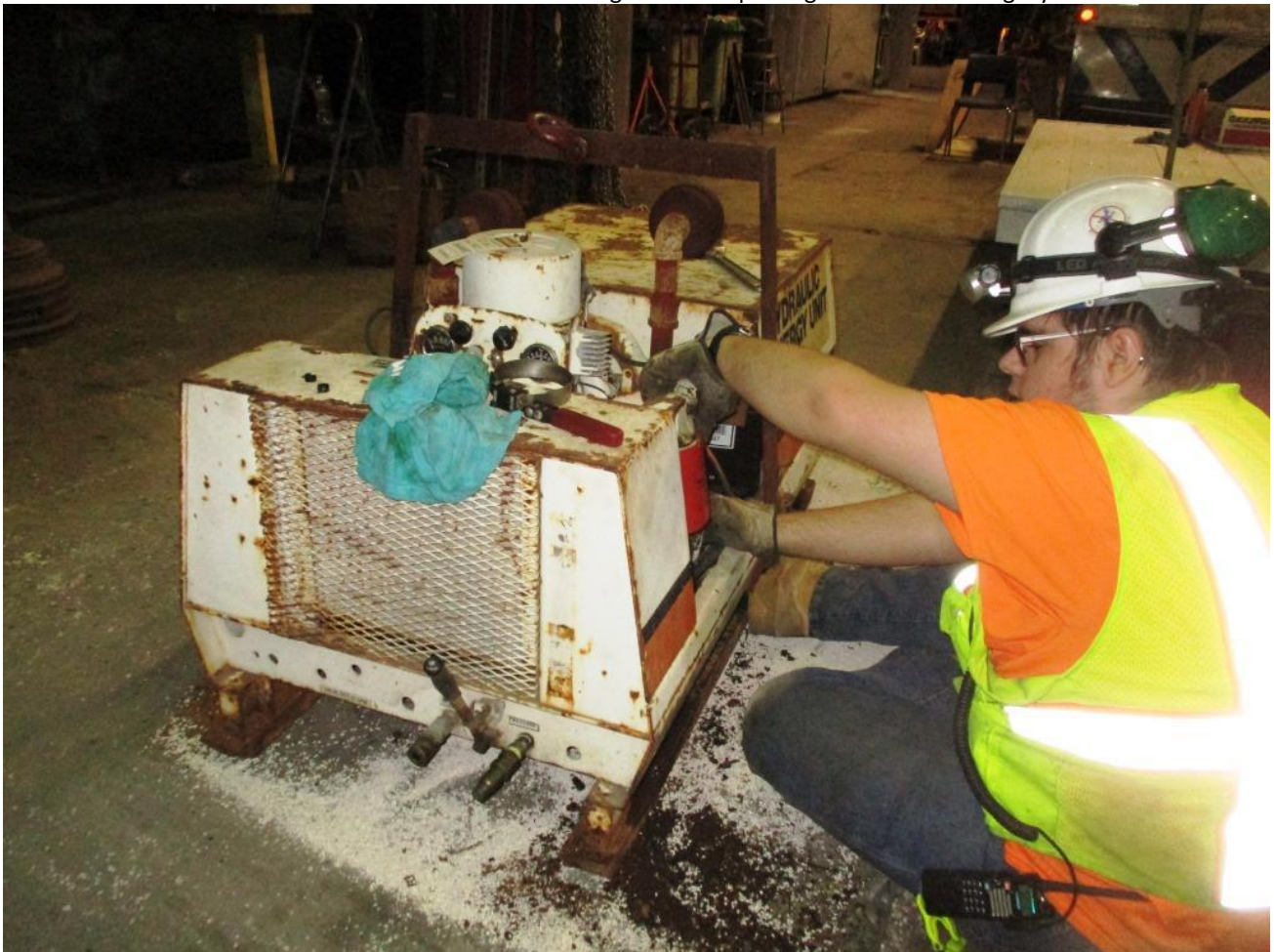
Chris H. installs a new filter on the hydraulic power unit
