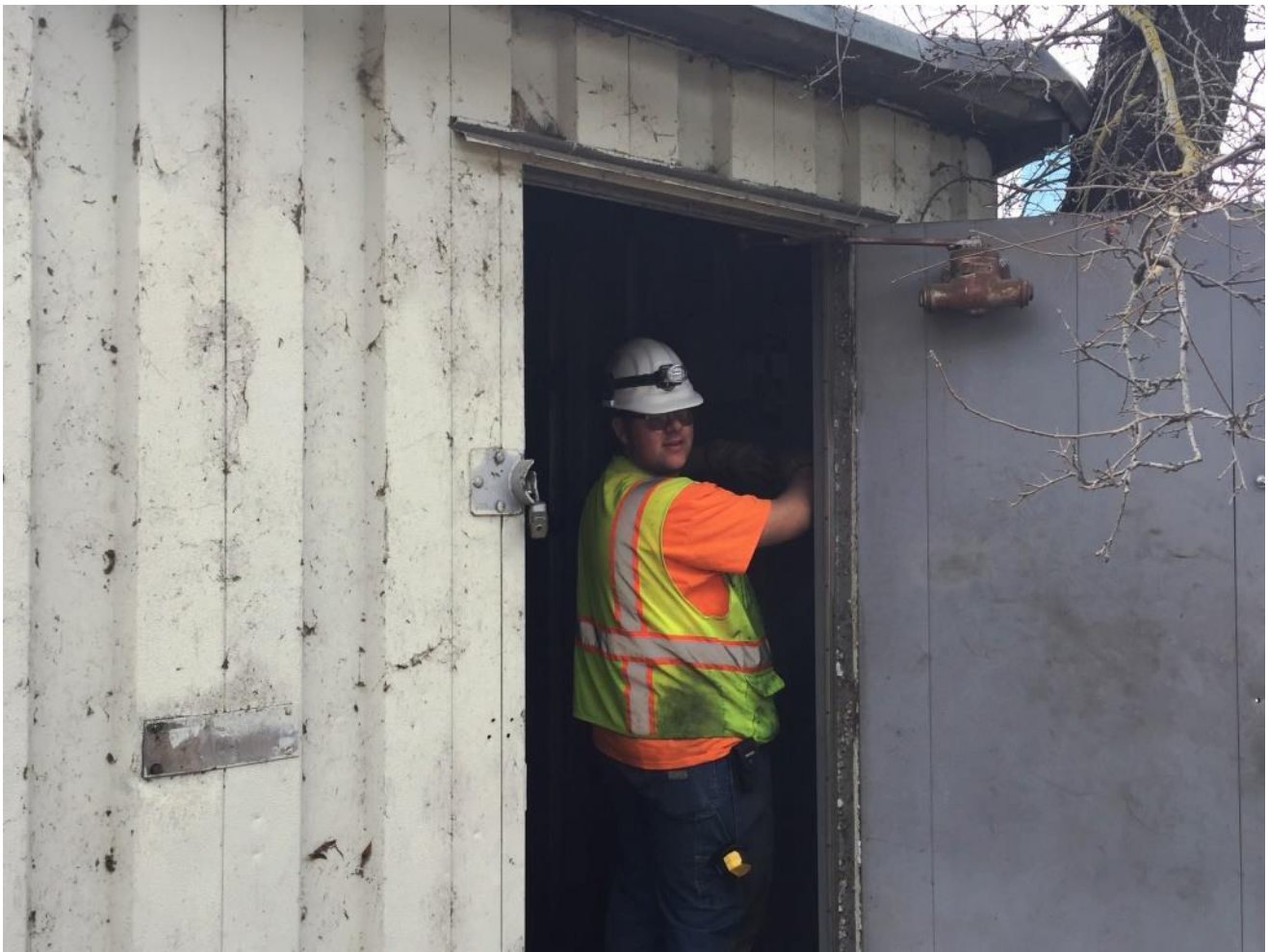
Meanwhile, Chris H. starts dismantling the interior of the aluminum shed which used to house electrical components for the I Street Bridge
