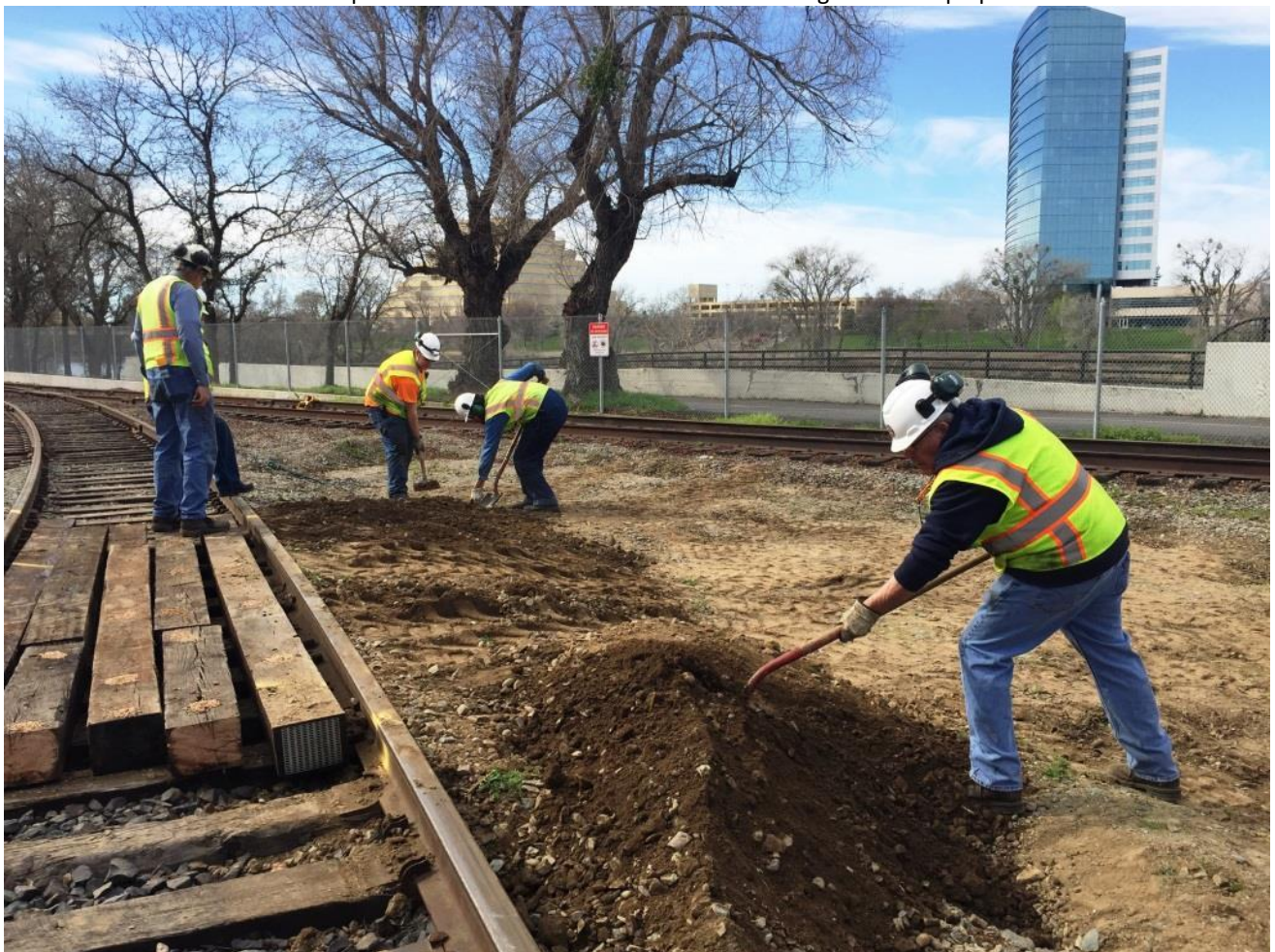
Bill, Chris H., and Weston spread the dirt being used to form a ramp
