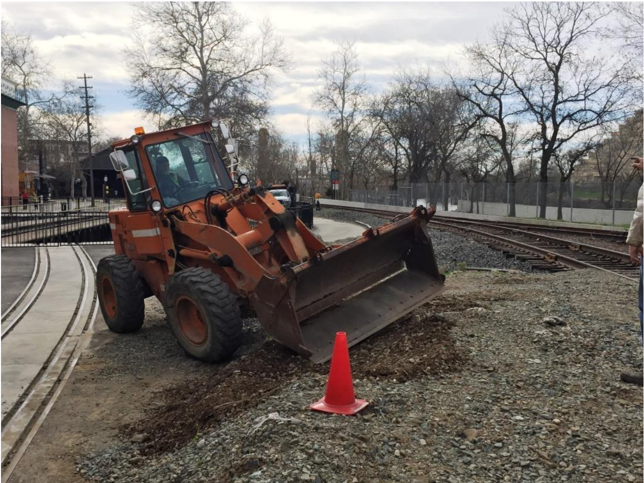
Mike F. in the loader building the ramp from the Whisker Track to the new crossing
