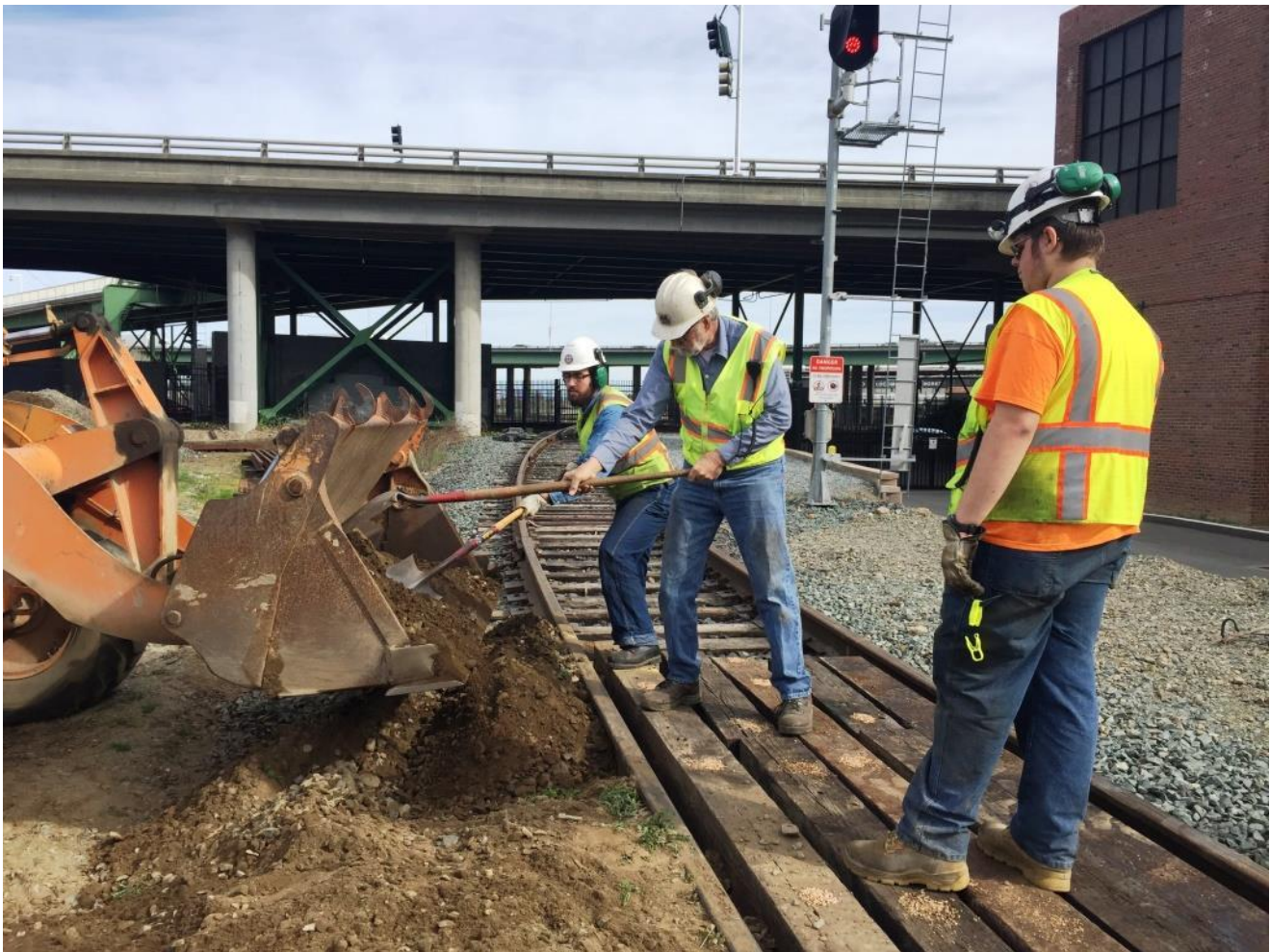
Weston and Alan scoop dirt from the loader's bucket in the building of the ramp up to the west rail
