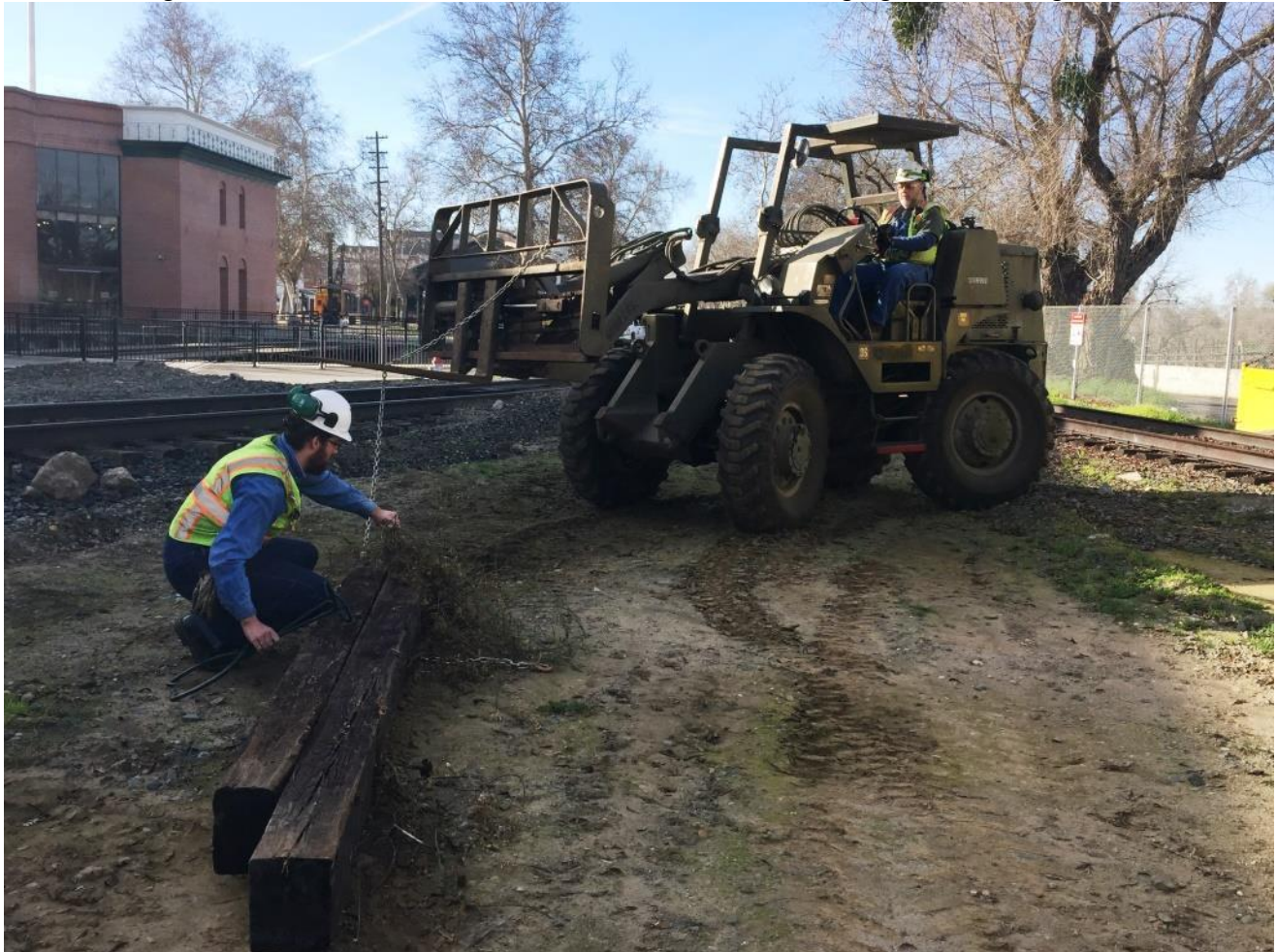
Weston attaches a chain to a tie which Mike F. on GM2 will pull into position
