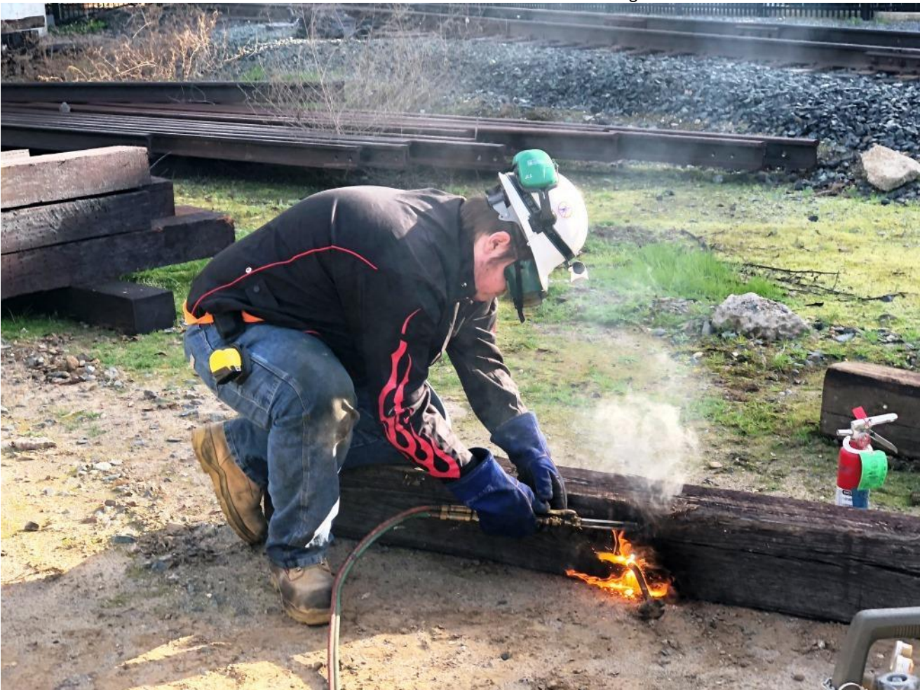
Chris H. torch-cuts a deeply embedded bent switch-bracket bolt off the tie
