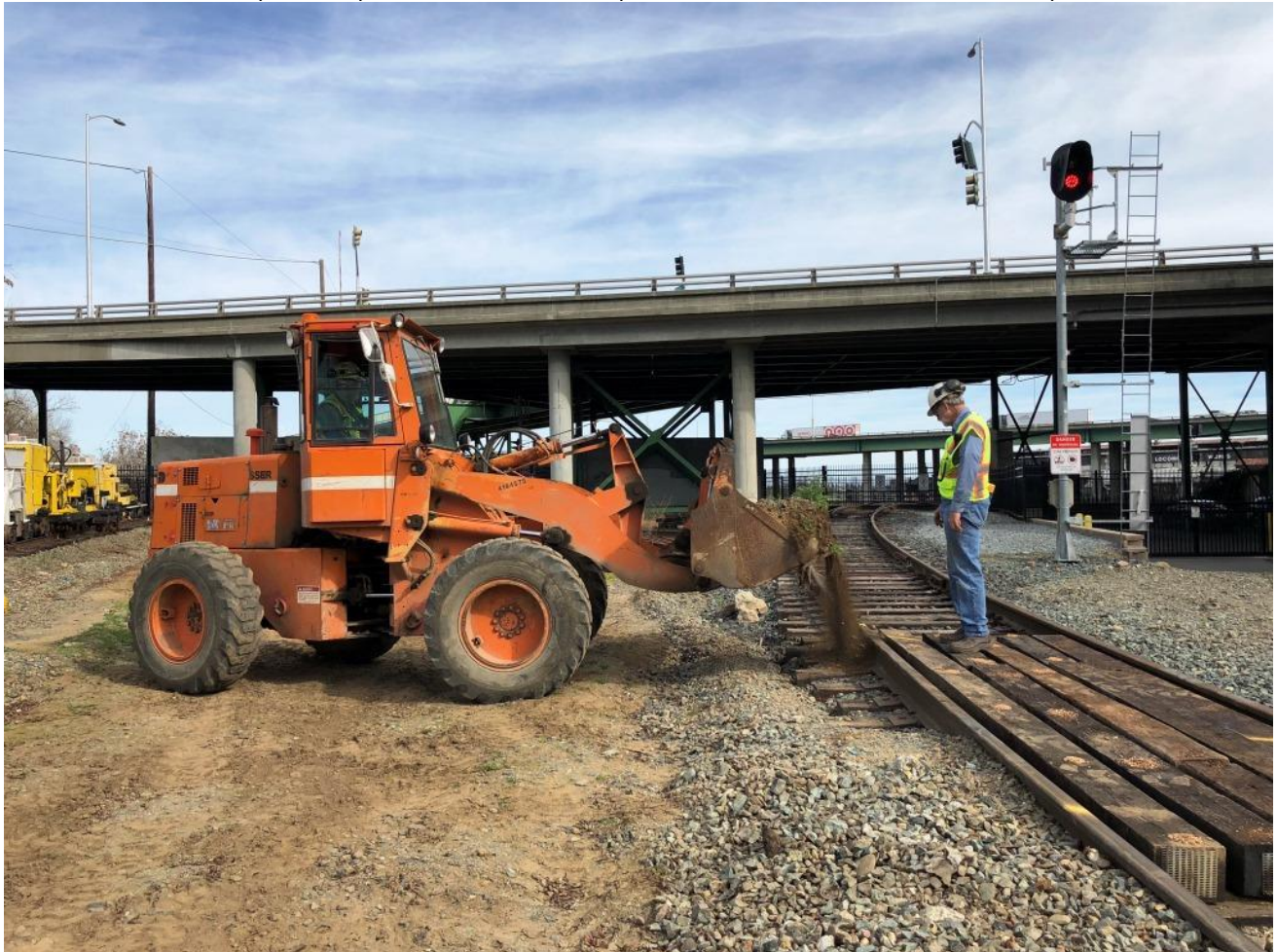
Alan guides Mike F., who brought the loader over to Old Sac., to start building ramps on each side of the 560 Track
