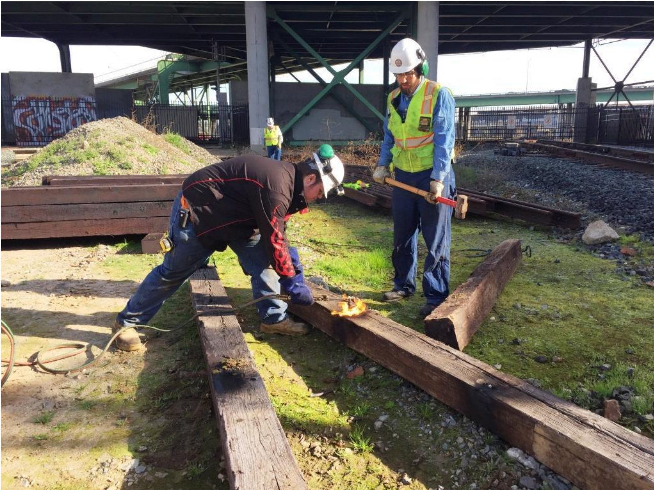
With a piece of the bracket-bolt still above the surface of the tie, Chris H. uses the torch to heat it up...
