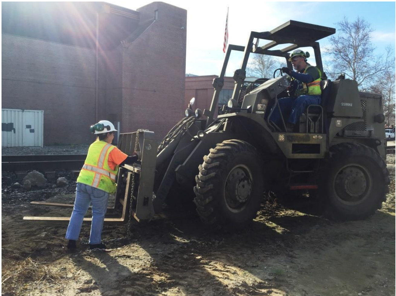
Pam connects the chain to GM2 which Mike F. will use to pull more ties from the pile
