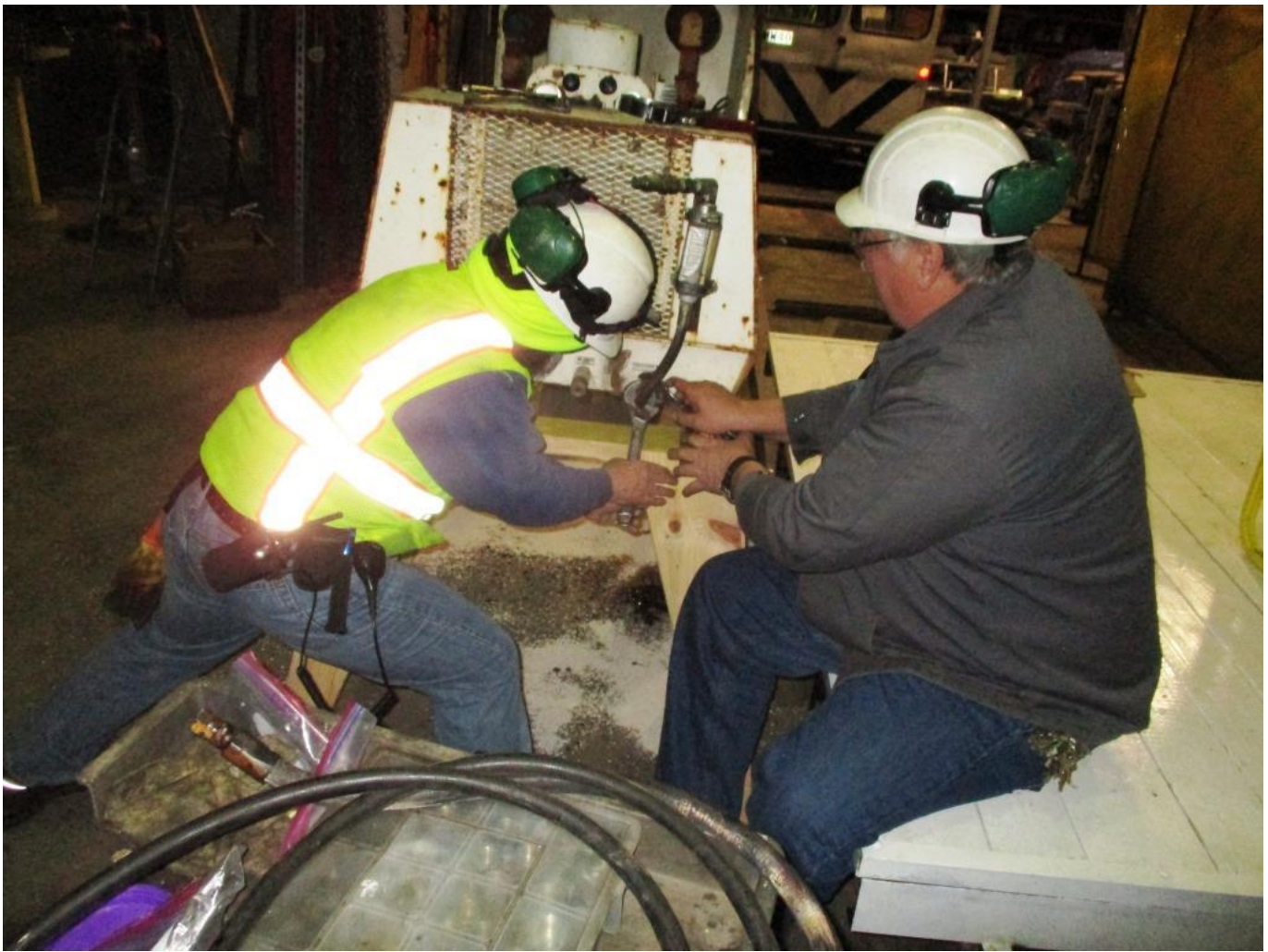
Joe and Chris C. repair "collision damage" to the hydraulic power unit
